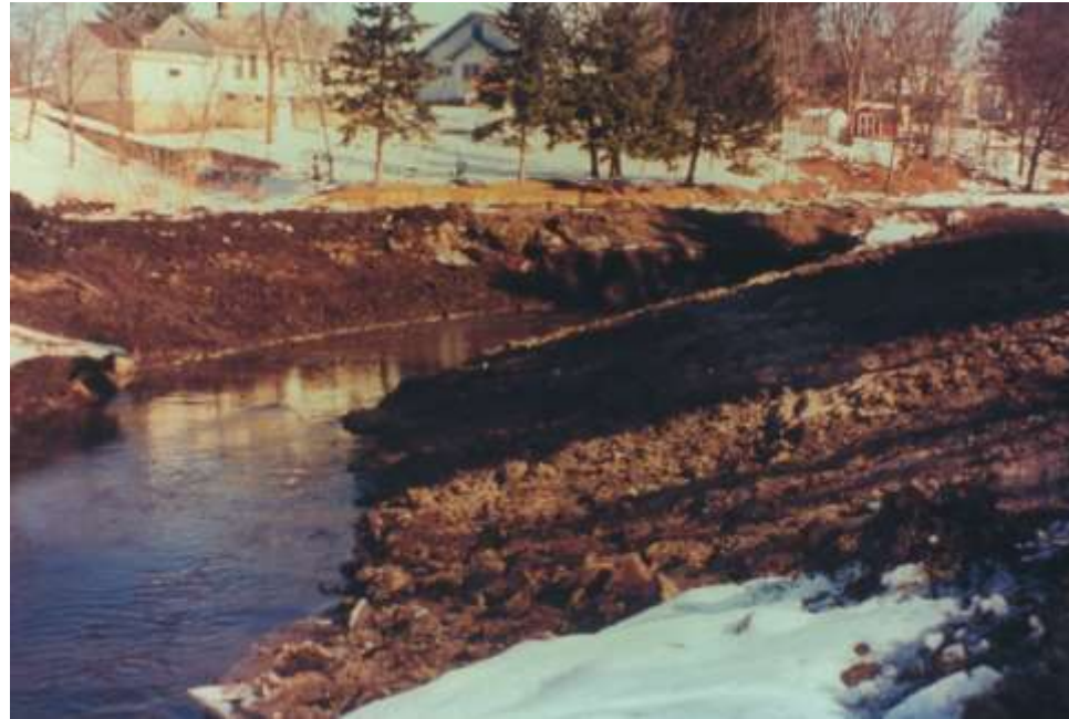
Former impoundment of Eighteen Mile Creek, immediately after removal
