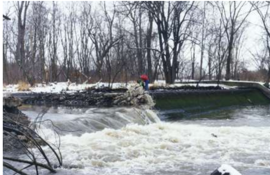
Waterworks Dam removal, Winter 97-98
